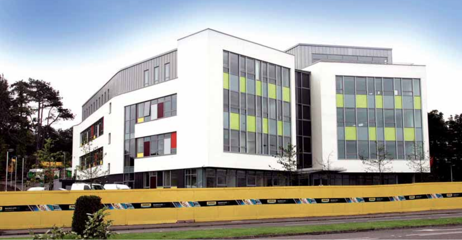
Knockbreda Wellbeing and Treatment Centre
