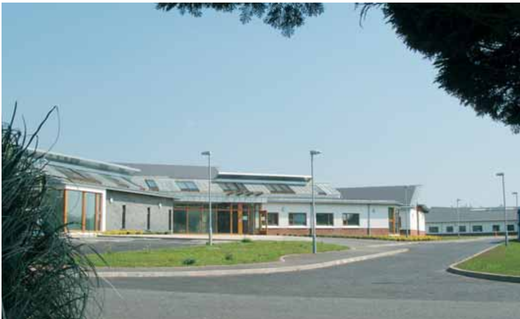
The new Cranfield Admission and Assessment Unit at Muckamore Abbey Hospital opened in October 2006
